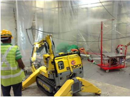
Fig.5 The misting machine (red machine on the right) being used in demolition works
