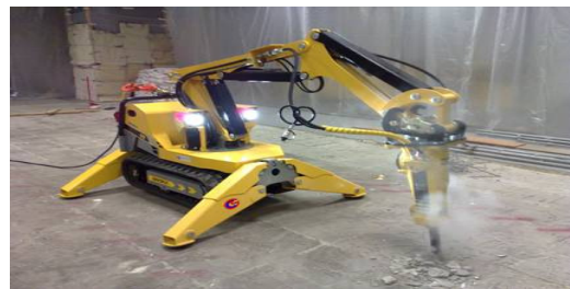
Fig.3 Demolition work being carried out
